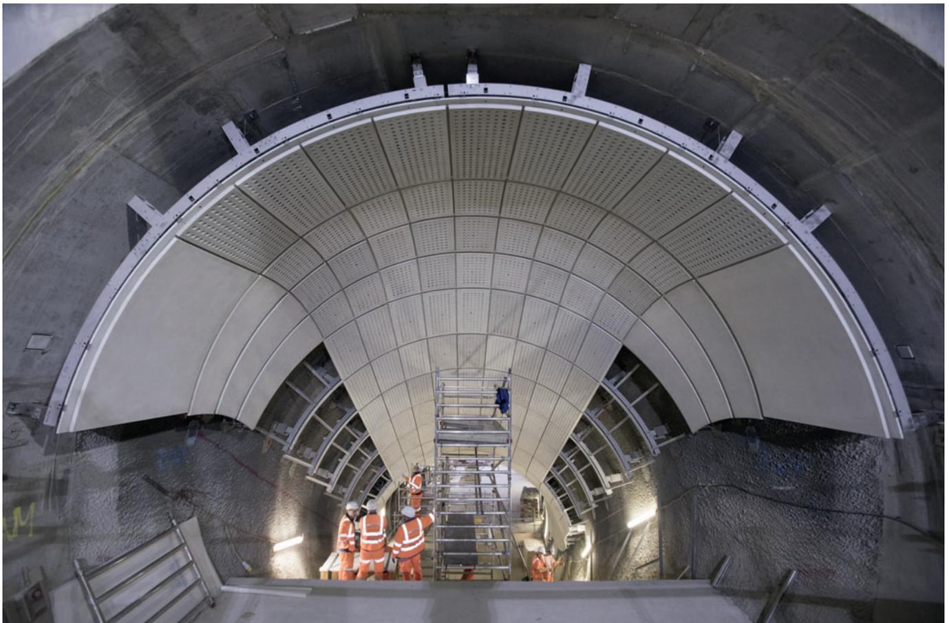
*The suspended façade panels are made from glass fibre reinforced concrete using the pressure spraying method.*
