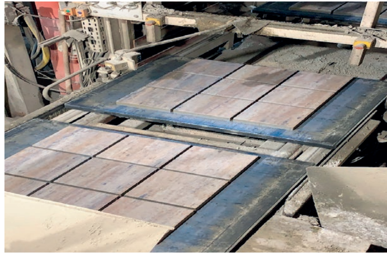
Wasa Uniplast Ultra in use at Betonwerk Huber in Altomünster
